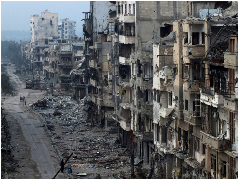
People stand on a street lined with damaged buildings in the besieged area of Homs January 27, 2014. Photo Yazan Homsy, Reuters.
