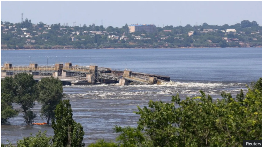
Ukraine's Kakhovka Dam after its destruction
